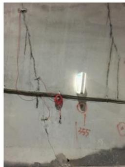
**Fig. 2.** Cracked lining
