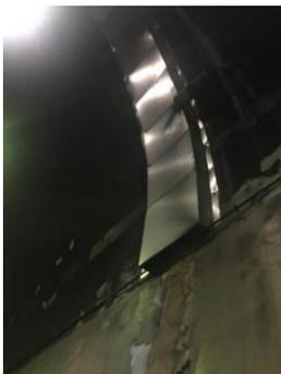
**Fig. 1.** Water box at a leak in the lining
