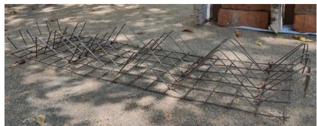
Fig. 3. Shear connector trusses tied with bottom wire mesh
