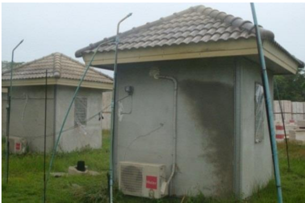
Fig. 2. View of the tested houses with the AAC and AAC with coated PCM wall materials
