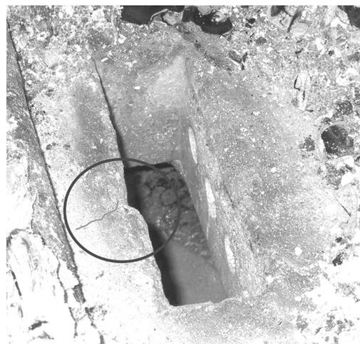
**Fig. 1.** Examples of castable products destruction in boiler (size  $(40 \times 20 \times 5) \text{ cm}$  and  $(60 \times 40 \times 10) \text{ cm}$ )
