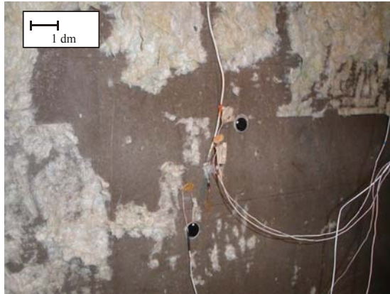
Fig. 4. Location of sensors on specimen for the determination of the thermal resistance
