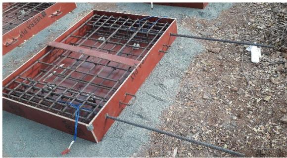
**Fig. 3.** Wall panel with protruding dowel bars
