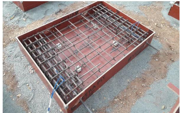
**Fig. 6.** Wall panel with protruding bars for coupler
