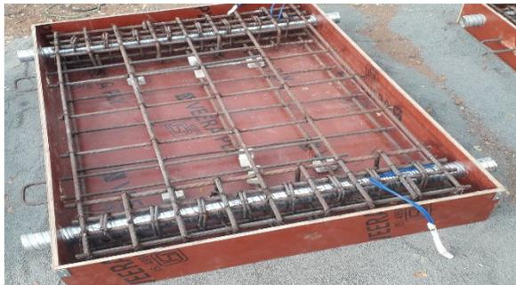
**Fig. 4.** Wall panel with grout sleeve
