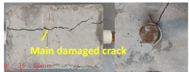
Fig. 4. Adhesion damage morphology
