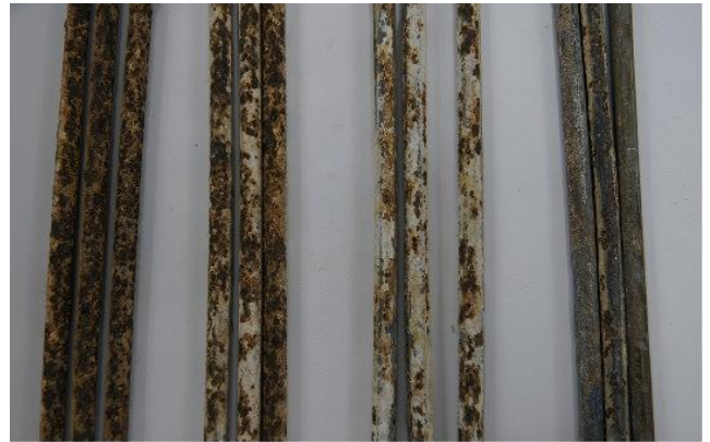
Fig. 9. Classification of corrosion severity in main cable steel wires
