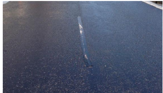
Fig. 12. Image after fog seal application
