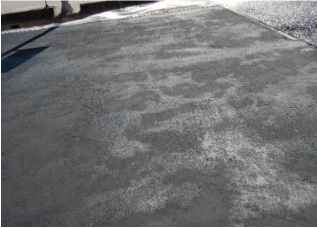
Fig. 13. Image after slurry seal application
